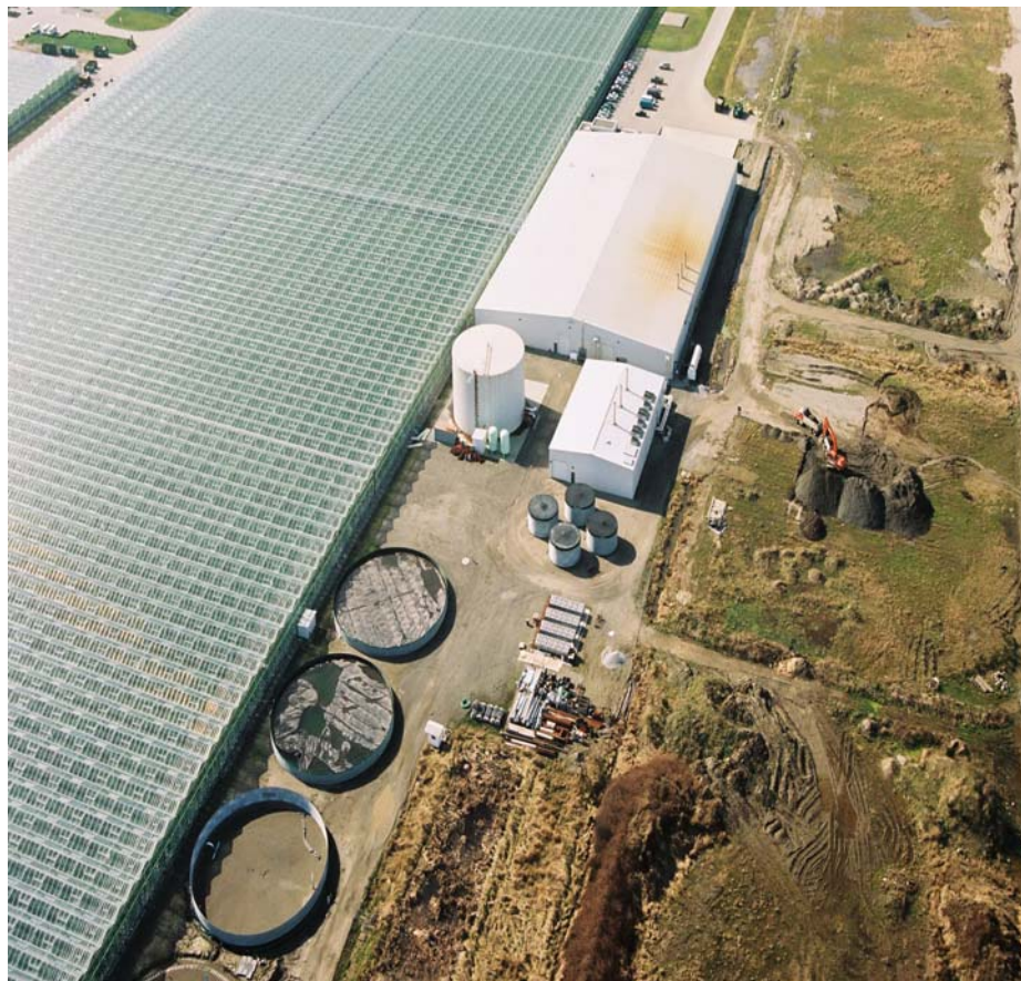
Greenhouse installations using landfill gas.
